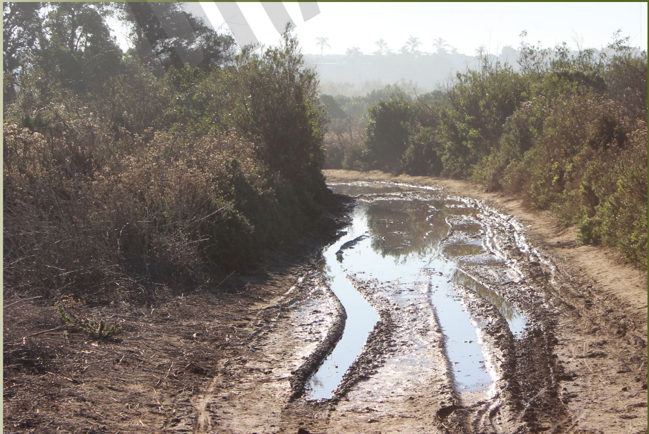
Trail improvements will correct existing conditions causing water to pool in low spots, enhancing emergency responsiveness and pedestrian access.
